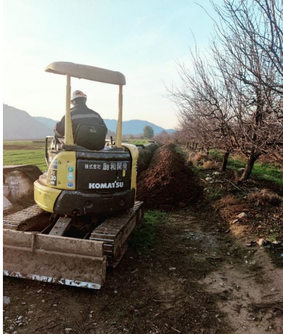
Image 3.D: Preparation for burying closed pump line for transporting manure to lagoon 2-5
