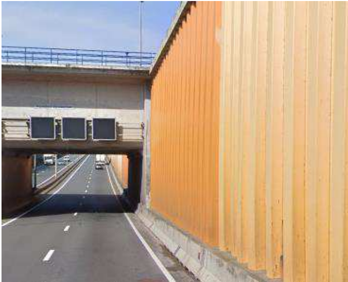
Figure 3.3 Rire-retardant coating on sheet piles
