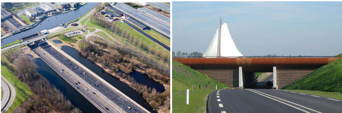
Figure 2.2 Large (left) and small aqueduct (right)
