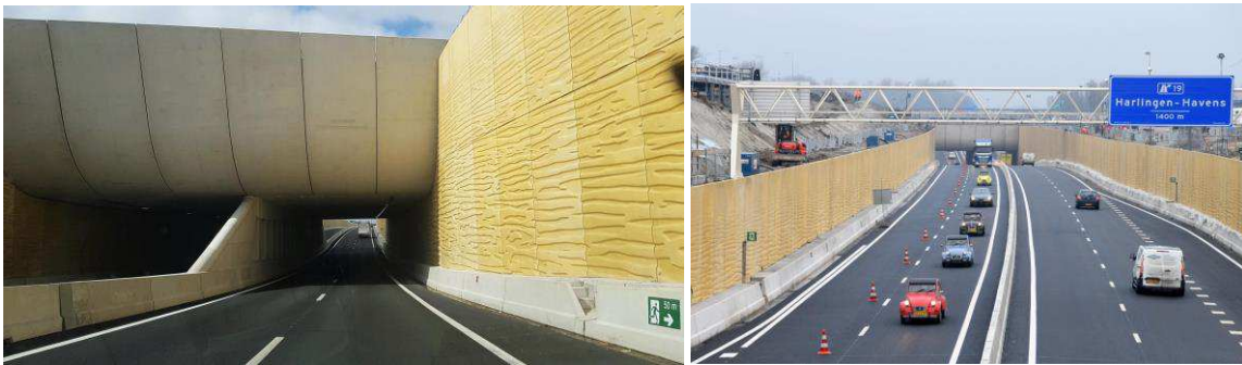
Figure 3.8 Photos of Van Harinxma aqueduct in Harlingen
