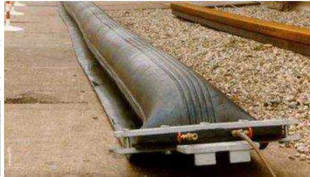
Figure 2.6 Inflated seal on construction site (right)
