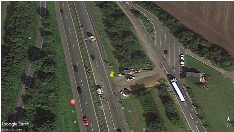
FIGURE 2.4. The measurement site at E45 a few hundred meters north of the Danish-German border. The yellow pin marks the position of the measurements
