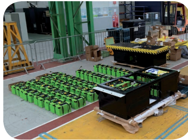
Batteries and assembly in one of six rafts
