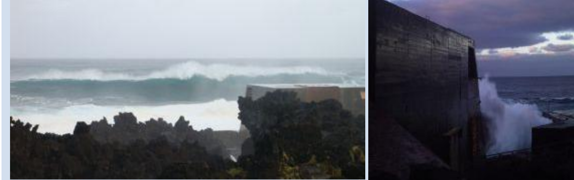
Pico Plant of 400 kW on the Azores in the middle of the Atlantic Ocean
