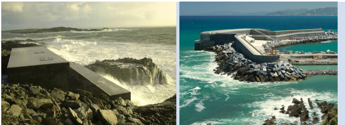
WaveGEN 500 kW, Islay UK Courtesy of Voith Hydro Wavegen Ltd.
