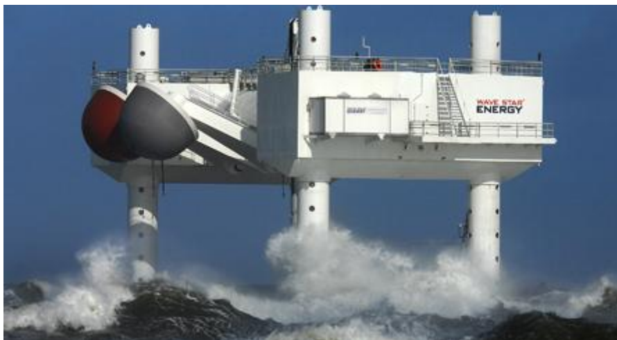
Figure 33 Wavestar investigates floaters of UHPC [w73]
