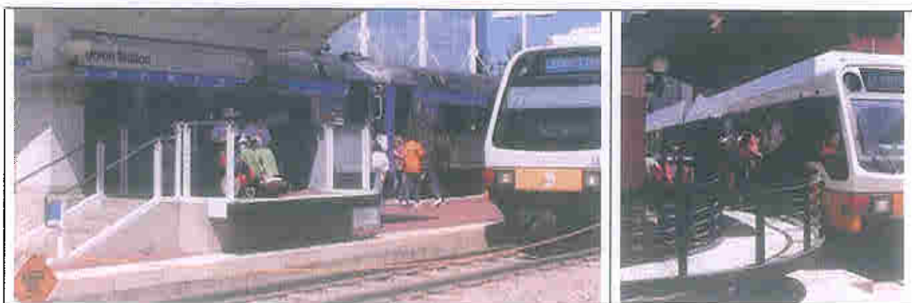
Graphic 1: fixed platform ramps (Dallas)
